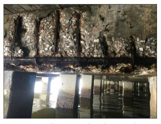
Figure 1-4: Berth 11. Severely Delaminated Concrete Pile Cap with Exposed Reinforcement
