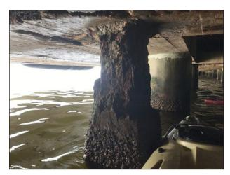
Figure 1-3: Berth 11. Severely Spalled Precast Concrete Pile
