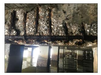
Figure 2: Berth 11. Severely Delaminated Concrete Pile Cap with Exposed Reinforcement
