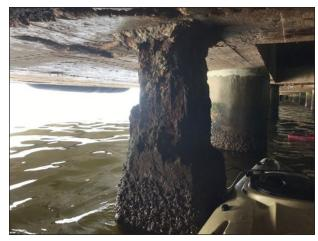
Figure 1: Berth 11. Severely Spalled Precast Concrete Pile
