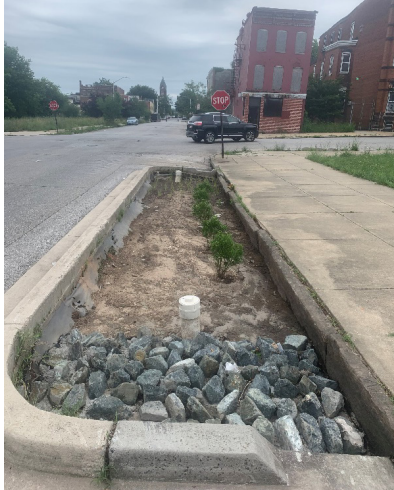
Figure 11: Example of a bioretention facility under construction by Baltimore City DPW
