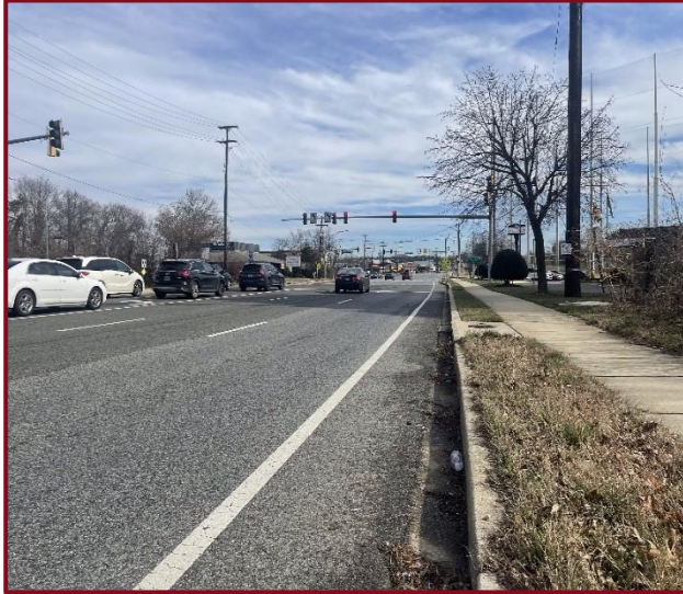
Figure 4. Bicycle Lane and Bus Stop on Oxon Hill Road
