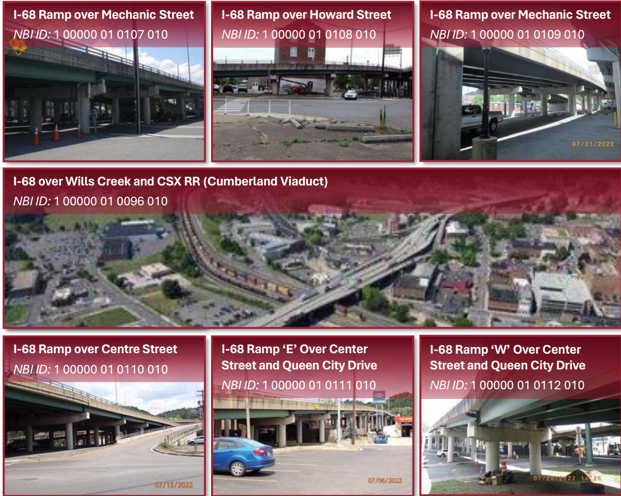
Figure 2-1 | Bridges in the Study Area
