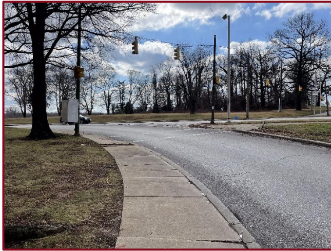
Figure 3. Existing Slip Lanes at Wabash Avenue and Patterson Avenue
