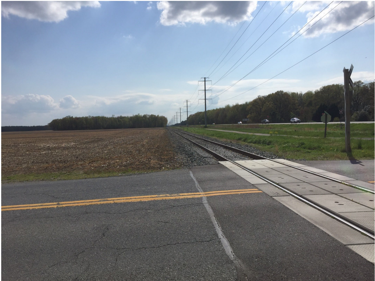
Figure 4-3. State-Owned Rail Line on Operated by Class II Railroad Maryland's Eastern Shore
