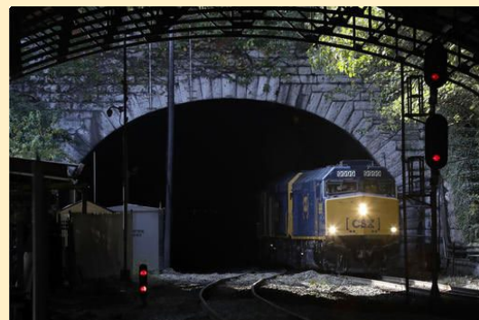
Howard Street Tunnel
