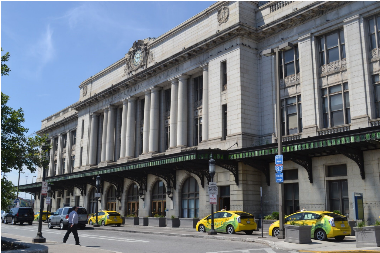
Figure 2-17. Baltimore Penn Station
