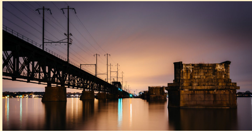
Bridge on Northeast Corridor North of Baltimore
