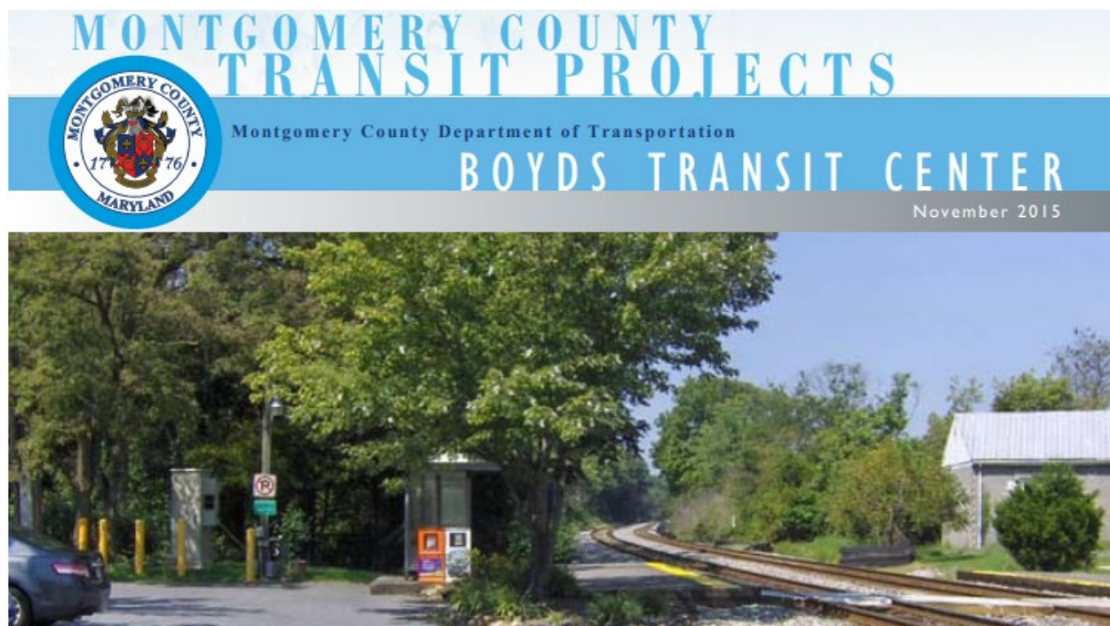
Figure 2-16. Boyds MARC Station
