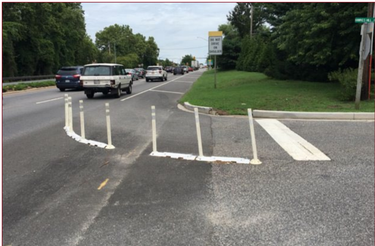
Figure 5. Current Condition with Plastic Delineators
