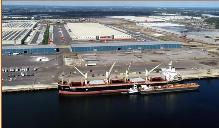
East Berth – Break Bulk Operation
