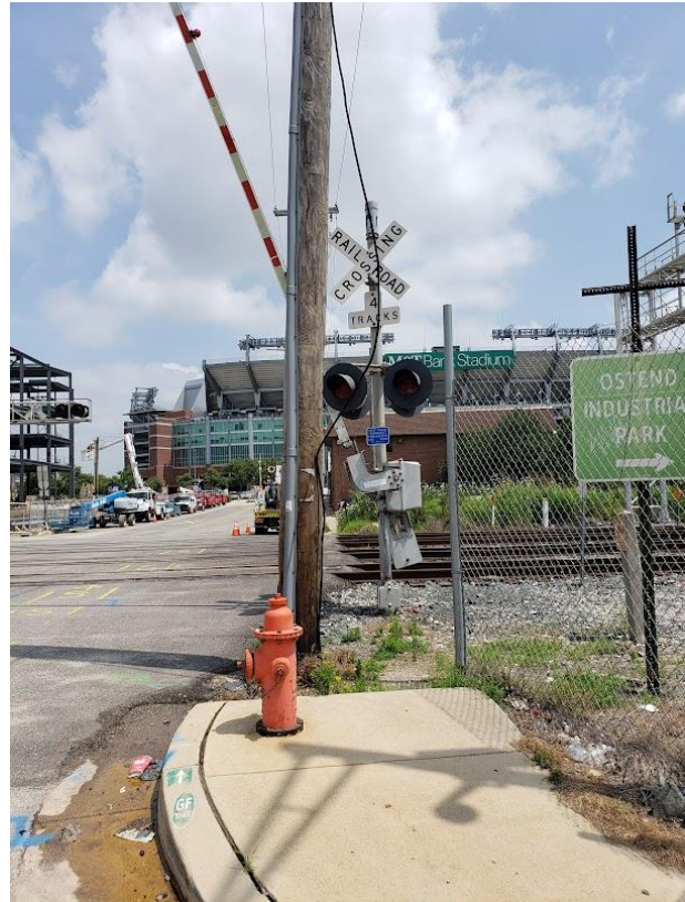
Figure 3: Existing conditions at Warner Street Rail Crossing
