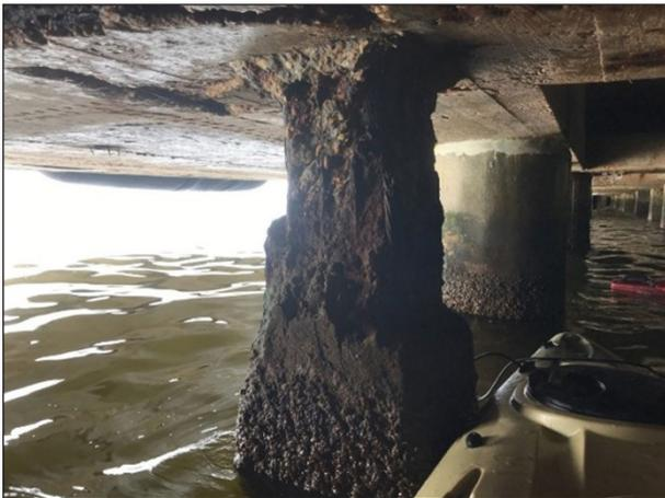
*Figure 1-3: Berth 11. Severely Spalled Precast Concrete Pile*
