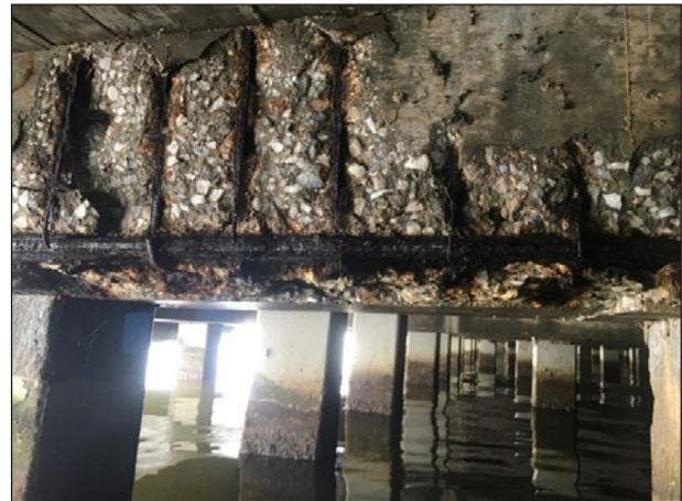
*Figure 1-4: Berth 11. Severely Delaminated Concrete Pile Cap with Exposed Reinforcement*
