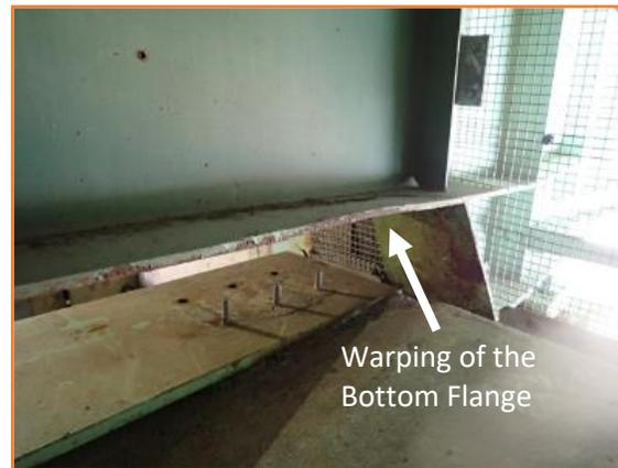
**Figure 44. Pack Rust between Bottom Flanges and Splice Plates**
