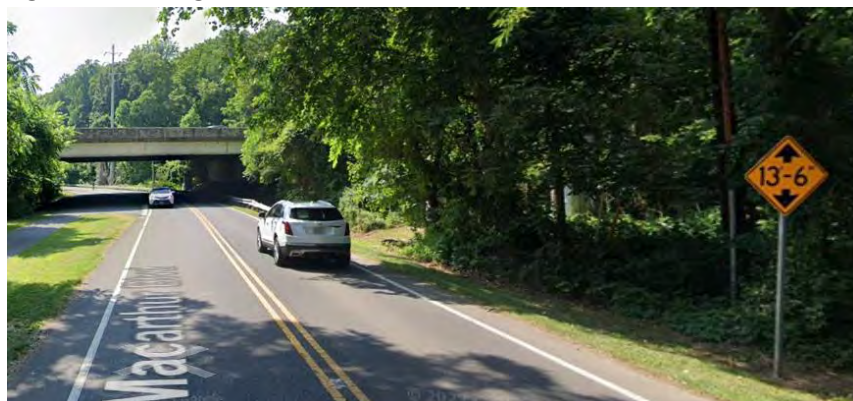
Figure 7. Existing Vertical Clearance - MacArthur Boulevard
