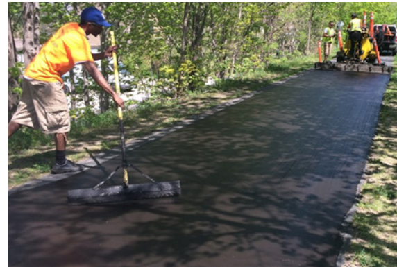
FIGURE 11 Preventative maintenance along an asphalt trail. (Source: Three Rivers Park District, Hennepin County, MN)
