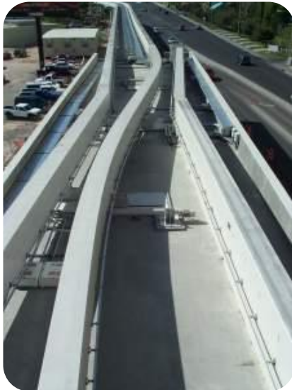
High speed beam replacement turn out switch
