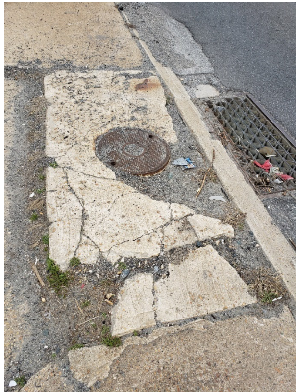
Figure 19. Sidewalks along US 1 in the Project Area in a State of Disrepair
