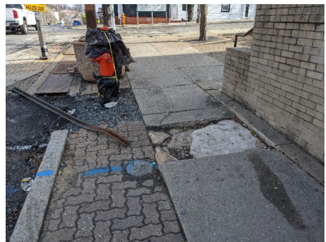
Figure 5. Sidewalks along US 1 The sidewalks along US 1 in the project area are in disrepair to the point of being impassable in places.
