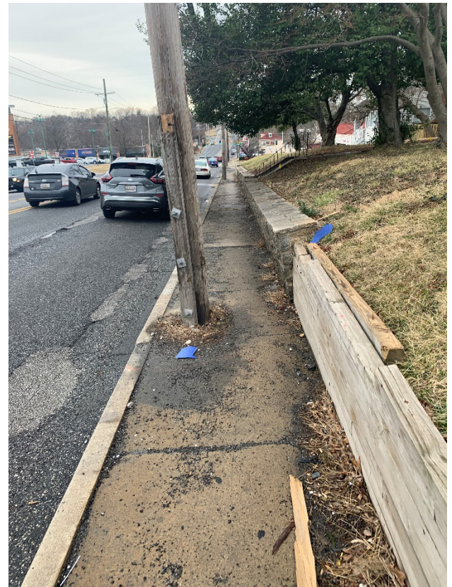
Figure 11 Narrow Sidewalks with Obstacles The sidewalks are narrow, blocked by utility poles, and bordered by retaining walls.
