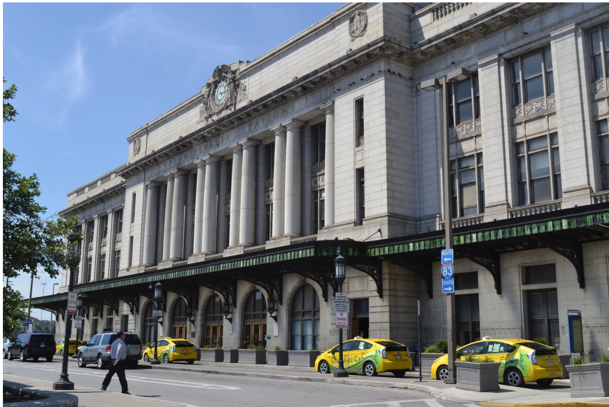
Figure 2-17. Baltimore Penn Station
