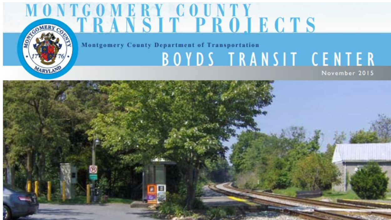
Figure 2-16. Boyds MARC Station
