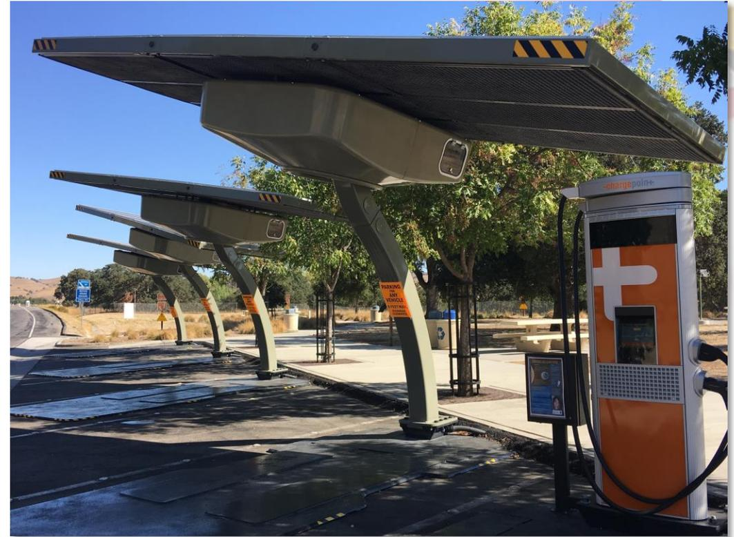
Fully solar-powered EV charging station deployed for CALtrans.
